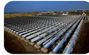
Solar Powered 500m3/day Seawater Desal Plant in Hawaii
